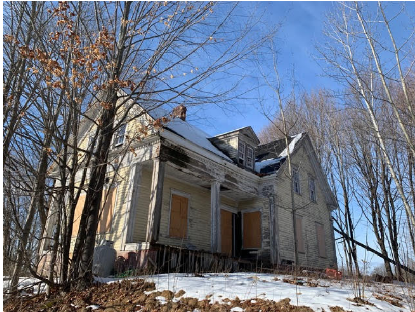
Condition of property when acquired in 2020.
